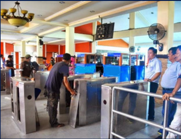
Install Tripod Turnstile for Ticketing Pass -PT. ASDP Indonesia
