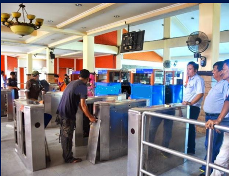
Install Tripod Turnstile for Ticketing Pass MRT Jakarta
